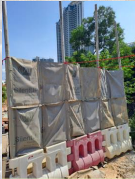
Deployment of noise barrier
