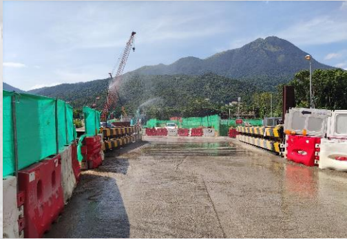
Water spraying via sprinklers at main access road
