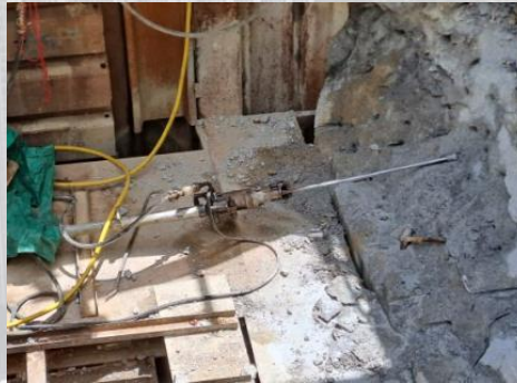
Concrete breaking by quieter method (Rock Splitter)
