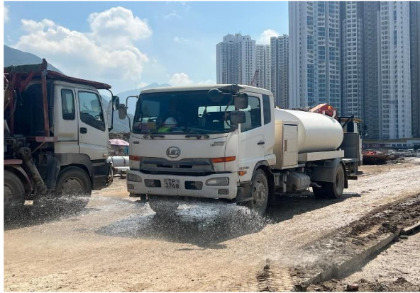
Water spraying by water truck for dust control
