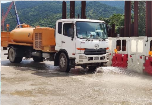
Water spraying by water truck along haul road
