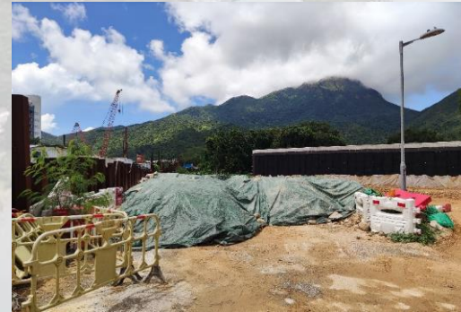
Covering excavated stockpiles by impervious sheeting
